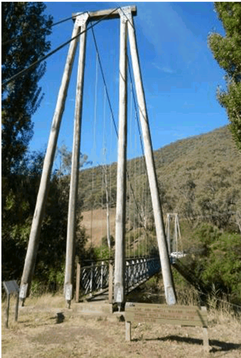
HUME AND HOVELL SWING BRIDGE OVER TUMUT RIVER
