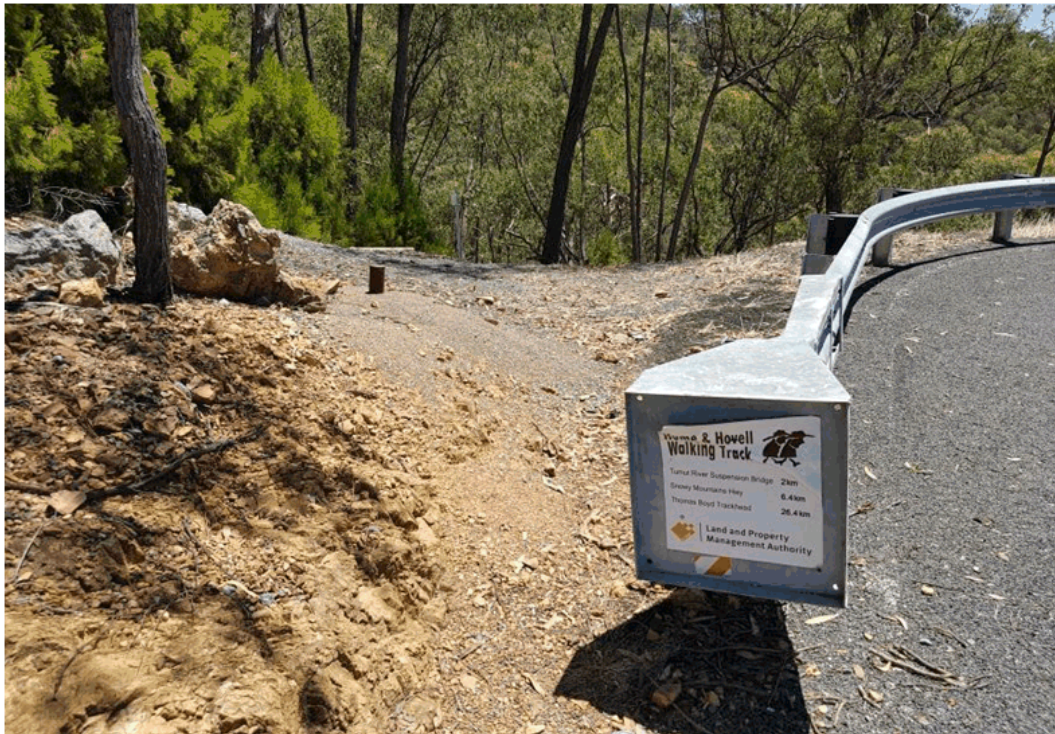
HUME AND HOVELL TRACK BLOWING DAM WALL
