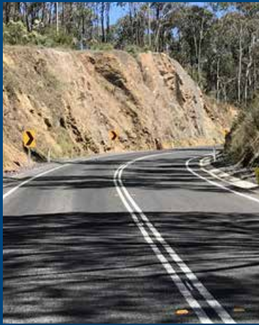
Final phase of Clarke's Hill reconstruction commences
