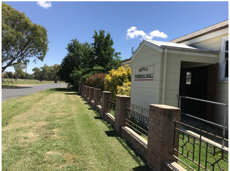
Figure 1 - Brungle Community Hall
