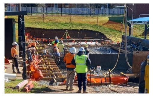
Works to replace the old baby and toddler pools with a learn-toswim pool and splash zone at the Tumut Pool complex is gaining momentum with teams recently completing a significant milestone of pouring the concrete for the learn-to-swim pool shell.
