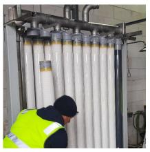
The membranes are made up of thousands of porous fibres that filter out various particles and impurities found in the raw water entering the plant.
