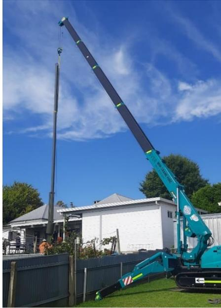
Many of the old concrete shafts are over 80 years old. When exposed to sewer gases concrete degrades making the vent shafts more susceptible to damage, lightning strikes and/or collapse, posing a danger to people and property.
