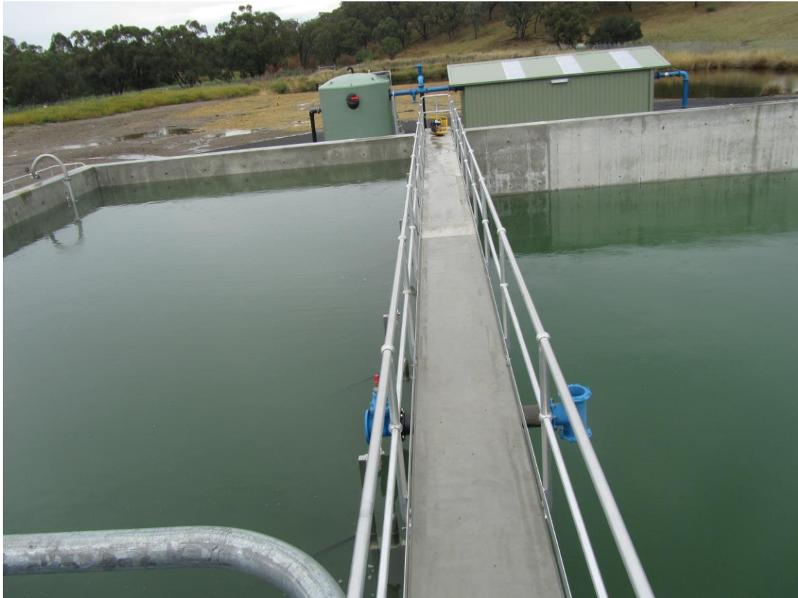
Figure 4.17 IDEA and Sludge Tank (right side)
