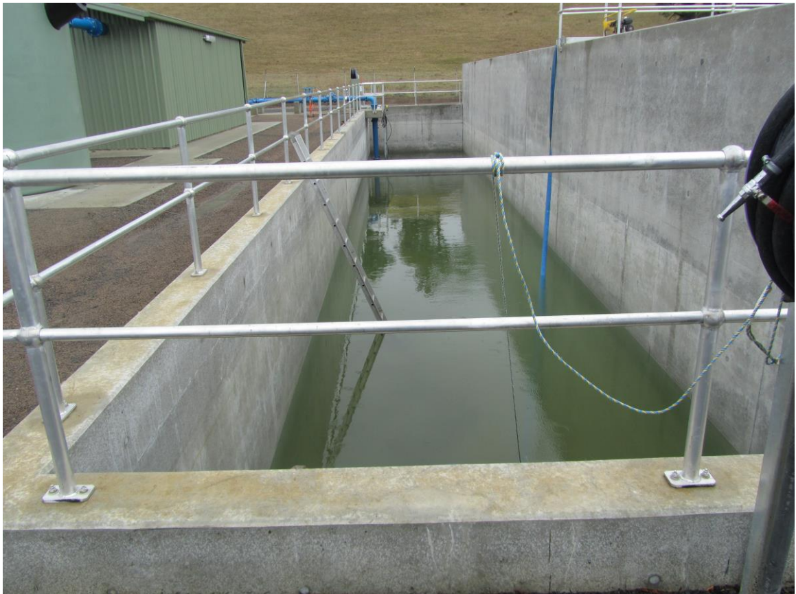
Figure 4.11 Balance Tank
