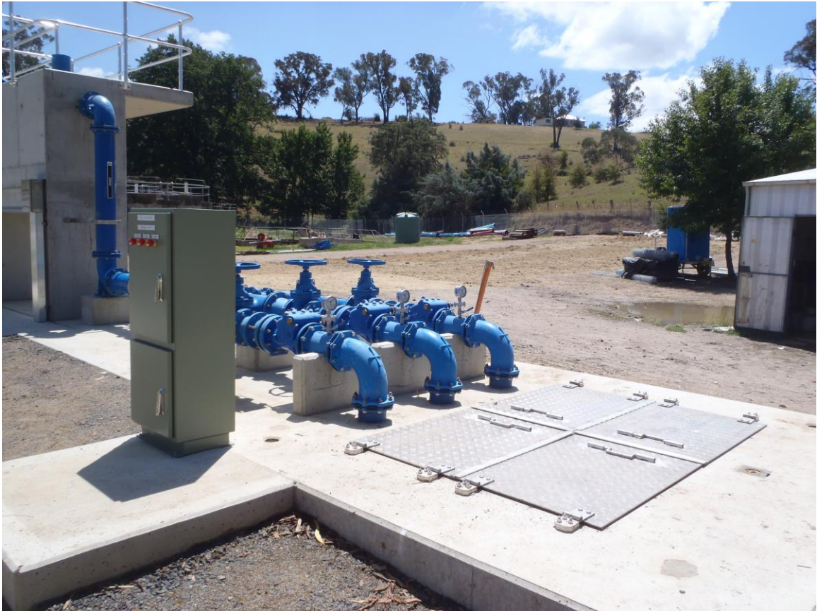
Figure 4.8 Inlet Works Lift PS
