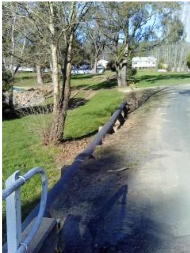
Figure 4.2 Exposed Sewage Pipeline without Barricade
