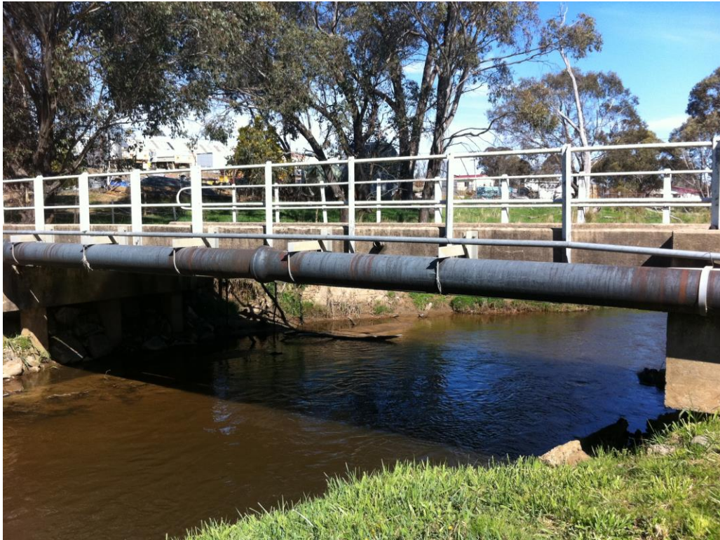
Figure 4.1 Sewage Pipeline Across Creek
