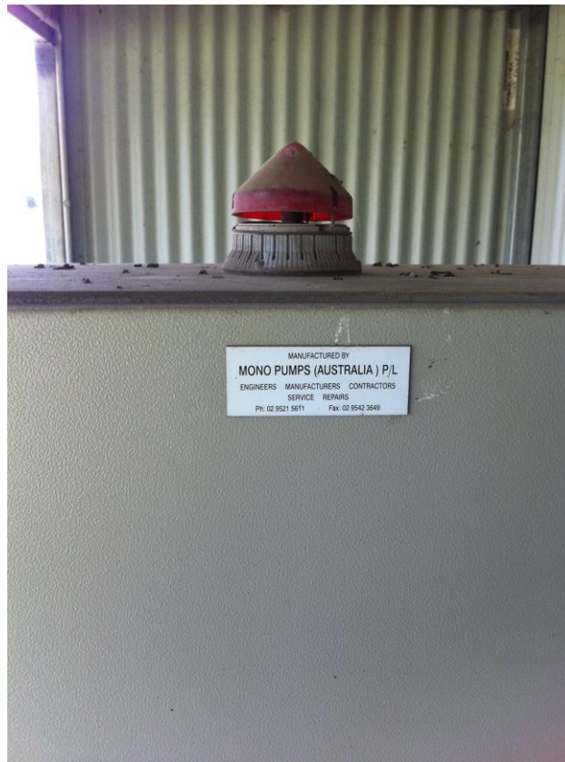
Figure 4.3 Alarm Light at HYNE MILL Pump Station
