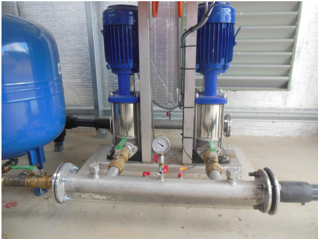
Figure 4.15 Onsite Reuse Pumps
