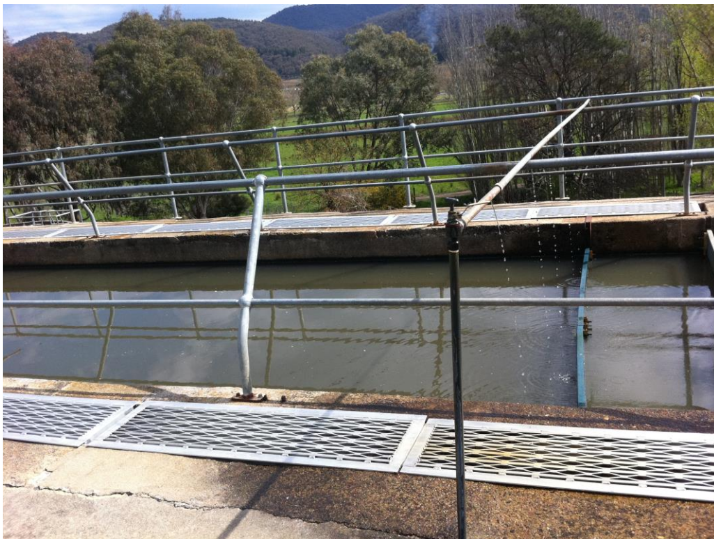
Figure 4.2 STP Sedimentation Tank
