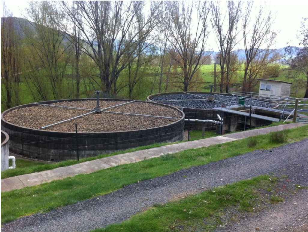
Figure 4.3 STP Trickling Filter Beds
