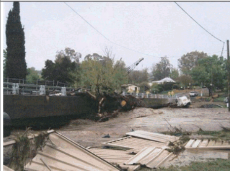
Plate 17 - View from No. 46 Tumut Street north towards partially constructed section of Herb Feint Bridge as flood recedes, shows accumulation of debris and influence in elevating water levels.
