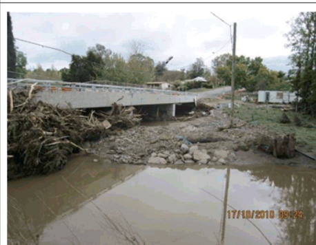
Plate 20 - Evidence of debris blockage on partially constructed section of Herb Feint Bridge, looking downstream.
