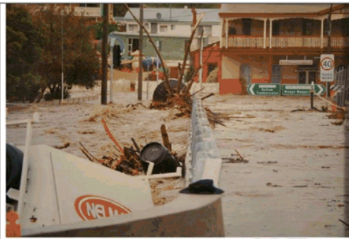
Plate 16 - View south across partially constructed section of Herb Feint Bridge, showing inundation of the bridge deck and debris trapped on upstream side.
