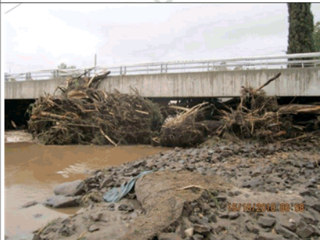
Plate 17 - View from No. 46 Tumut Street north towards partially constructed section of Herb Feint Bridge as flood recedes, shows accumulation of debris and influence in elevating water levels.
