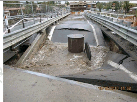
Plate 18 - Middle section of the remaining downstream half-width of Adelong Bridge collapsed.
