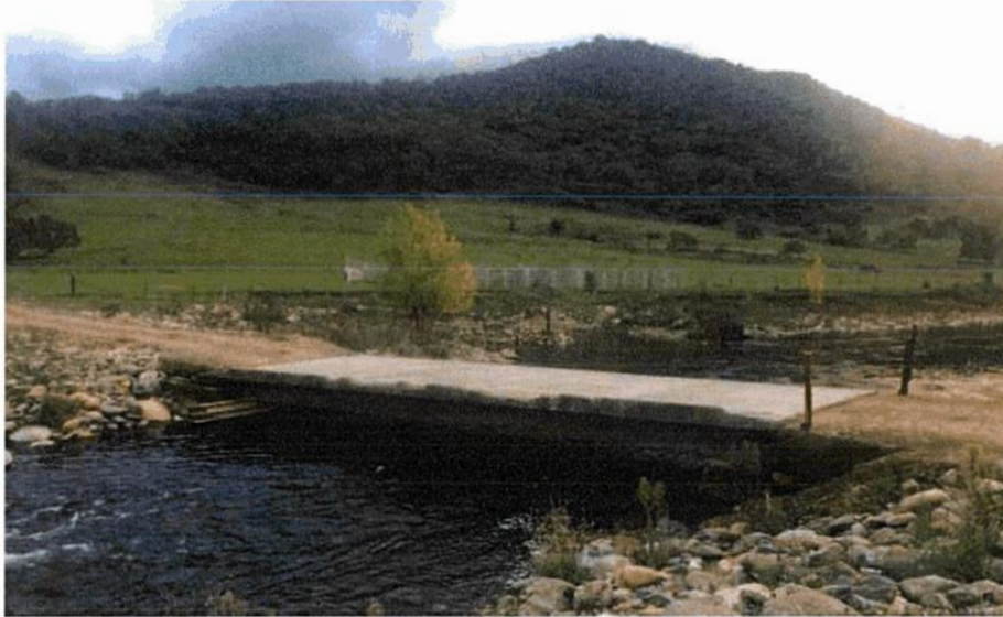
Photo 3 – Indicates the steel and concrete bridge that crosses the Goobarragandra River to allow access to the subject site (Bradley Cameron 2019).
