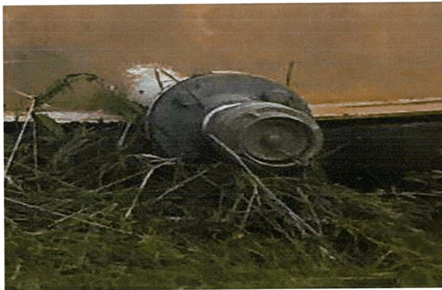
Photo 8 -Indicates the 65mm Storz coupling on one of the 20,000L water tanks located adjacent to the existing shed on the subject Lot (Bradley Cameron 2019)
