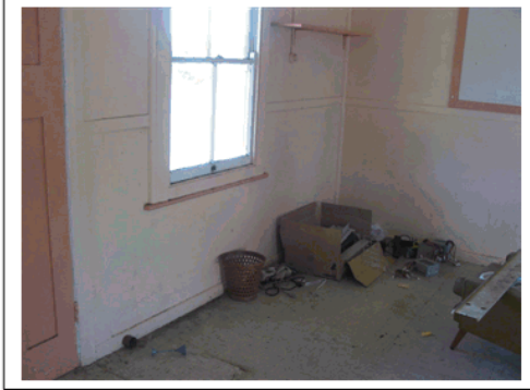
Plate 9: Display Centre – Internal wall sheet
