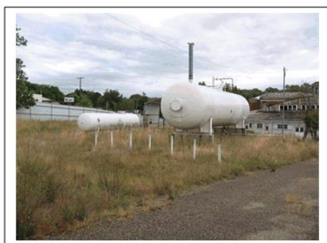
Plate 32 . LPG Gas Storage South of C & D Building
