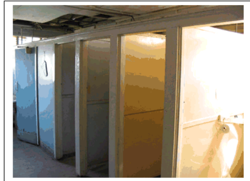
Plate 12: Cannery – West Offices – Asbestos Partitions to toilets
