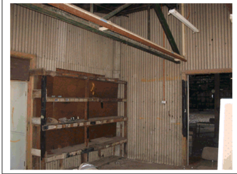
Plate 5: C & D Building – Asbestos Corrugated Wall Sheet
