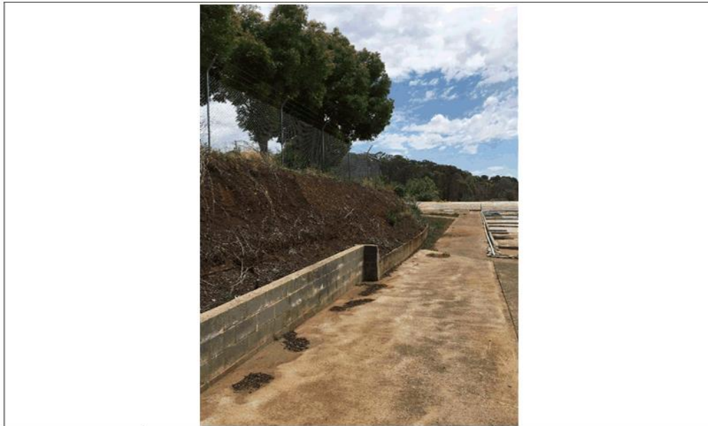
Photograph 15 Date: 1/12/2020 Evidence of cutting into natural soil to level the site along the west boundary of the site. View to the north.
