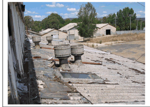
Plate 6: C & D Building: Asbestos Corrugated Roof Sheet, South end.
