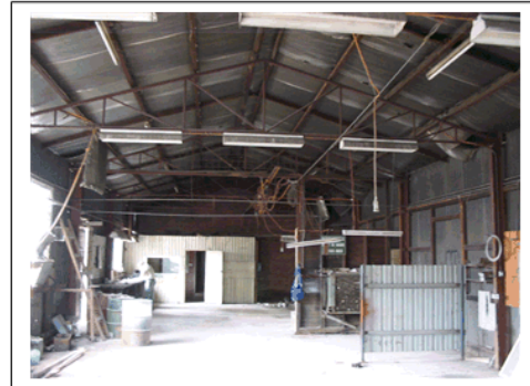
Plate 20 : Assume Fibre glass insulation to roof in Cannery Building
