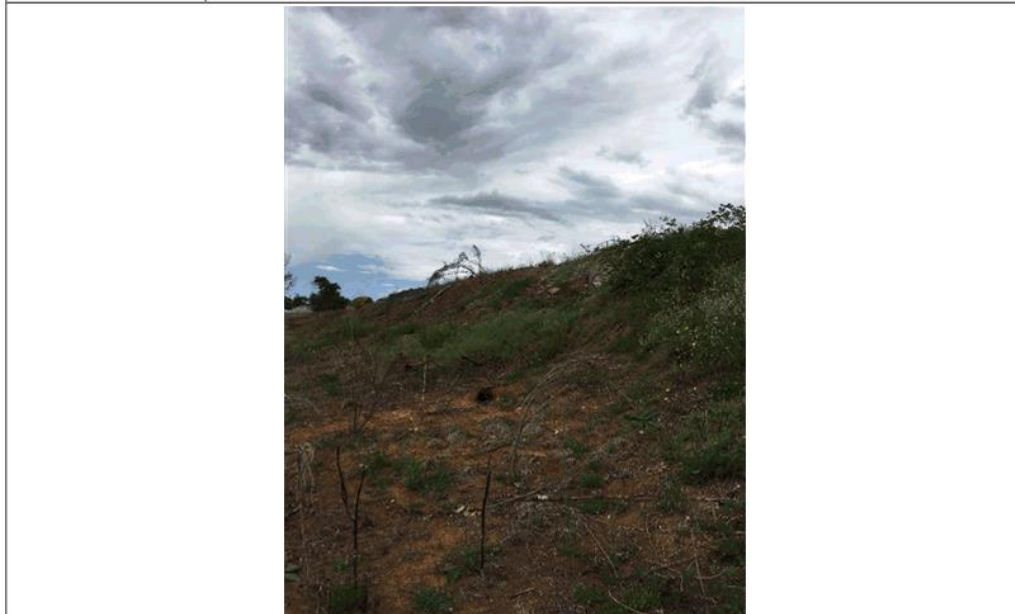
Photograph 16 Date: 1/12/2020 Evidence of backfilling to level site along the east boundary of the site. View to the southwest.
