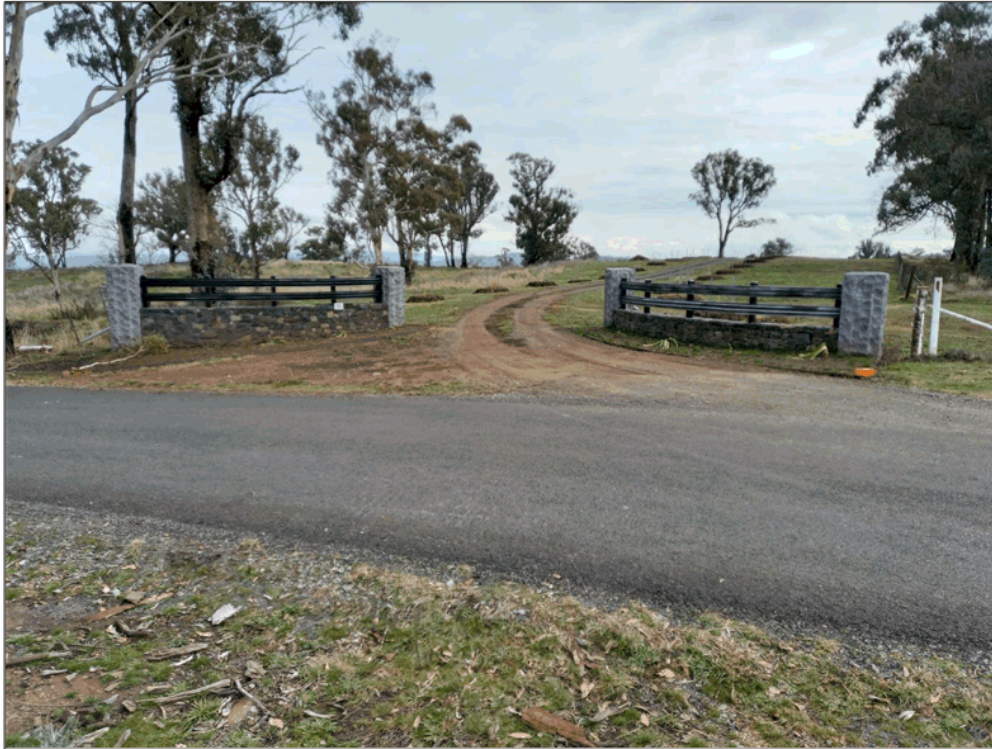
Figure 3: Existing Property Access via Paddys River Falls Road
