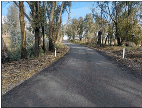
(a) View south
