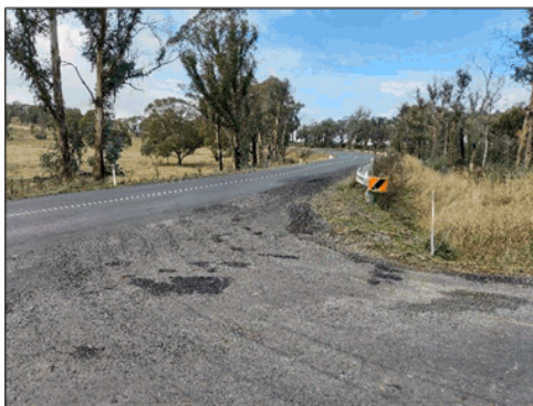
(a) View east
