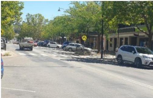
Figure 3-17 Faded marking (Capper Street / Richmond Street intersection)
