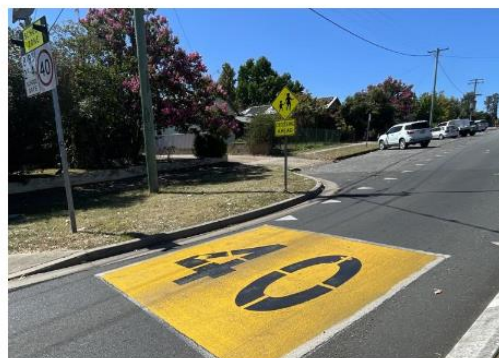
Figure 3-19 40km/h speed zone and dragon's teeth marking (Snowy Valleys School, Capper Street)
