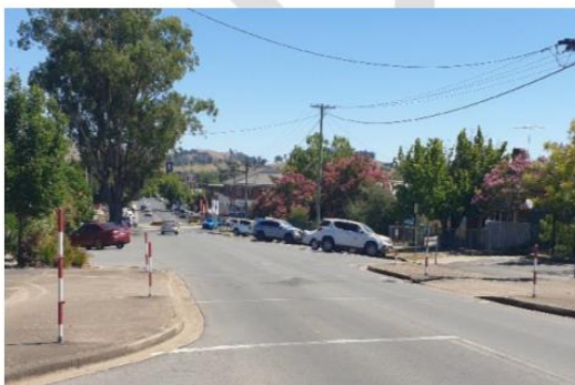
Figure 3-7 Faded Children's Crossing at Snowy Valleys School (Capper Street)
