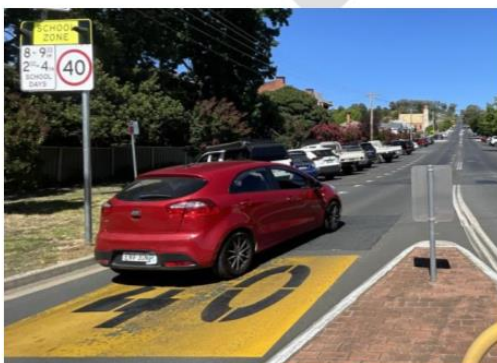
Figure 3-18 40km/h speed zone and dragon's teeth marking (Tumut Public School, Wynyard Street)
