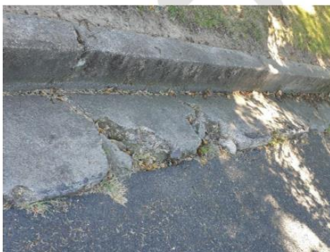
Figure 3-22 Damaged Kerb (Richmond Street)
