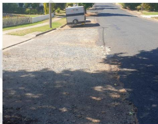
Figure 3-21 Exposed Road (Simpson Street)
