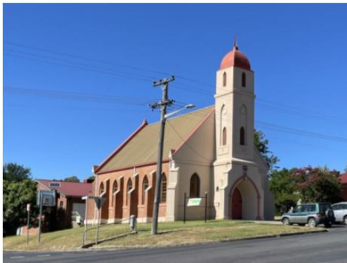
Figure 3-10 No kerb ramp at St Stephen’s Uniting Church (Simpson Street / Wynyard Street)
