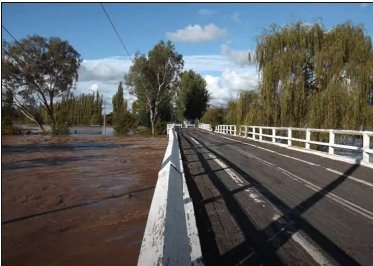
Figure 6: Flooding in the Bombowlee Avenue Locality 2012 – Old Tumut Bridge
