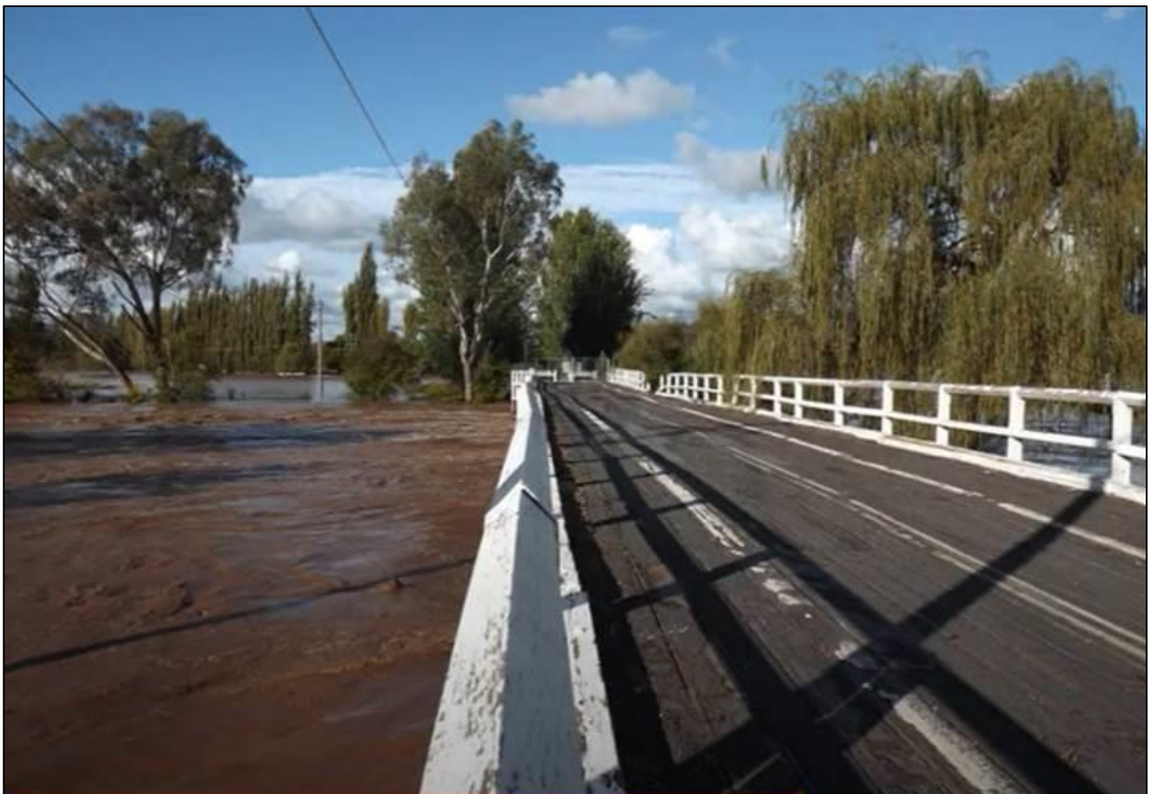
Figure 2: Flooding in the Bombowlee Avenue Locality 2012 – Old Tumut Bridge
