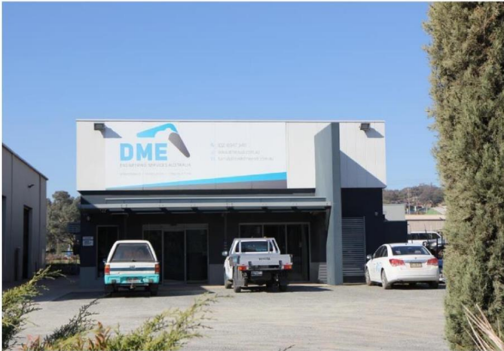
Photograph 14 – Location of accessible industrial car parking
