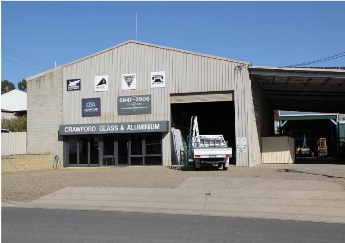
Photograph 15 – Signage relevant to the activity and size of the building
