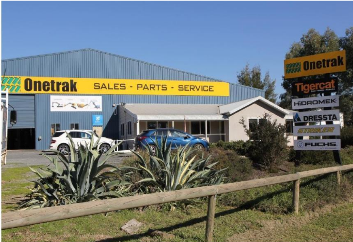
Photograph 12 – Office location at the front entry to the building and site
