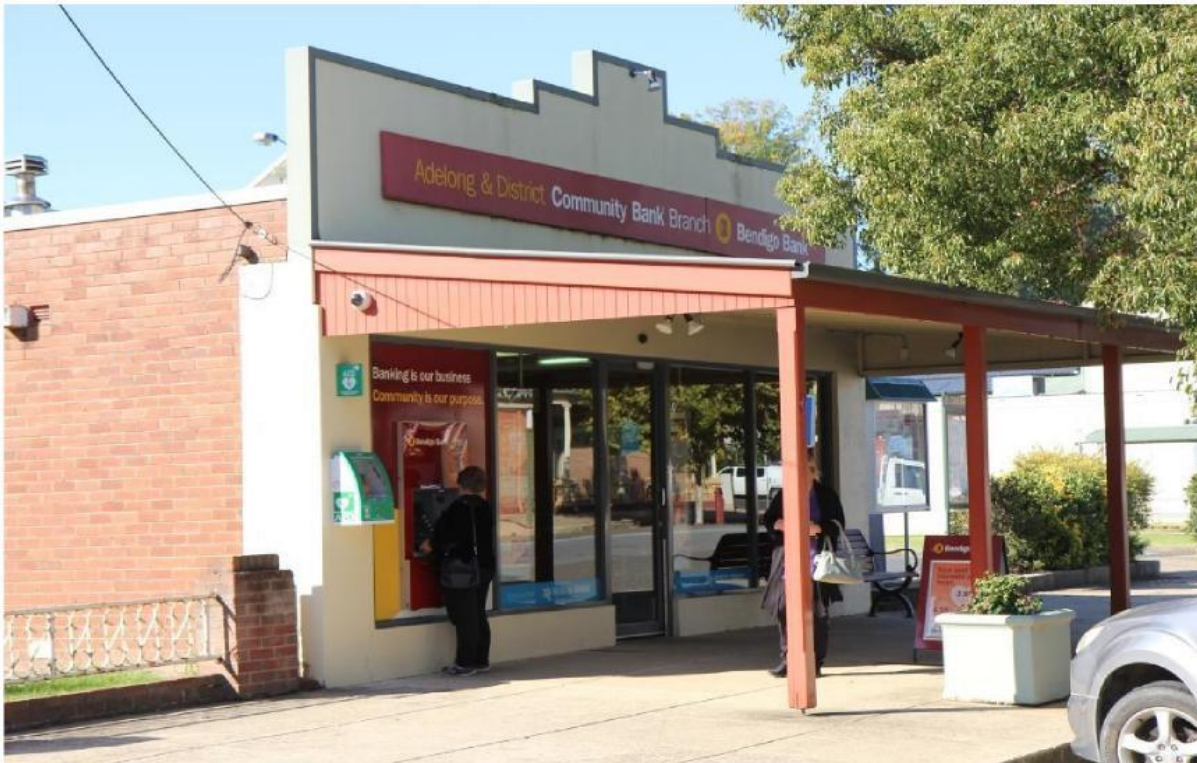
Photograph 1 – Commercial development and building design addressing the streetscape
