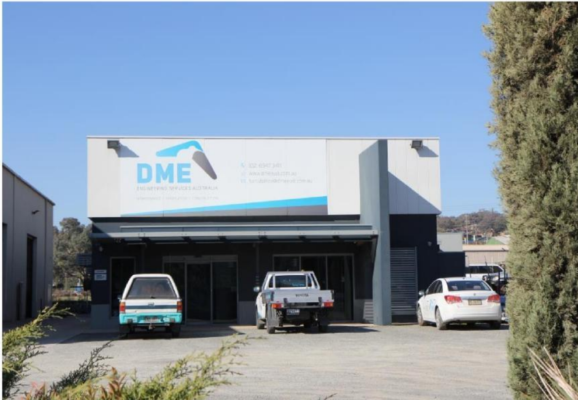
Photograph 14 – Location of accessible industrial car parking
