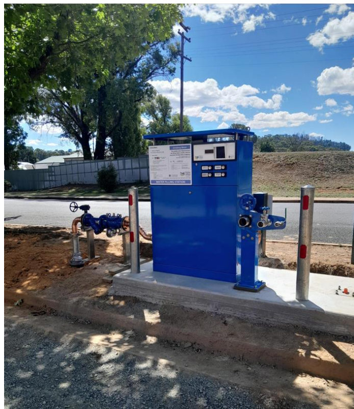
Image 2 - New Batlow Potable Water filling station installed at Memorial Avenue – Batlow - February 2025
