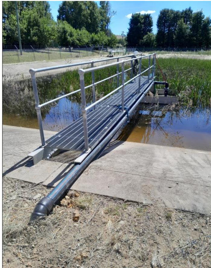
Image 3 - New Adelong Pipe Work for raw water filling station at - Todds Road - Adelong - completed February 2025
