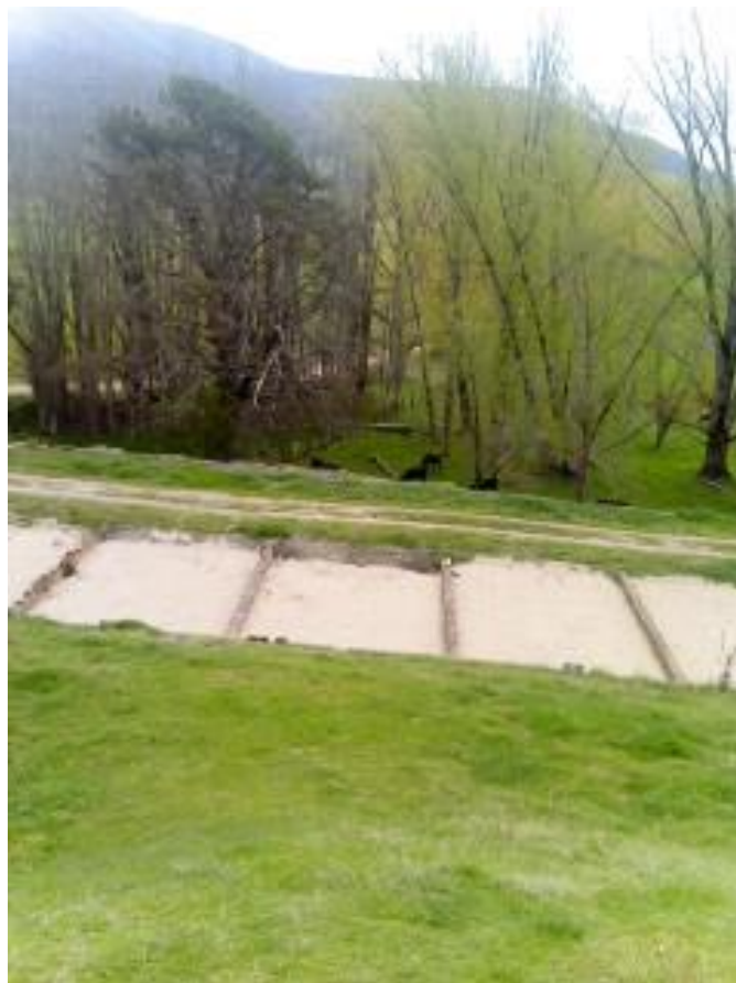
Figure 4.6 STP Sludge Drying Beds
