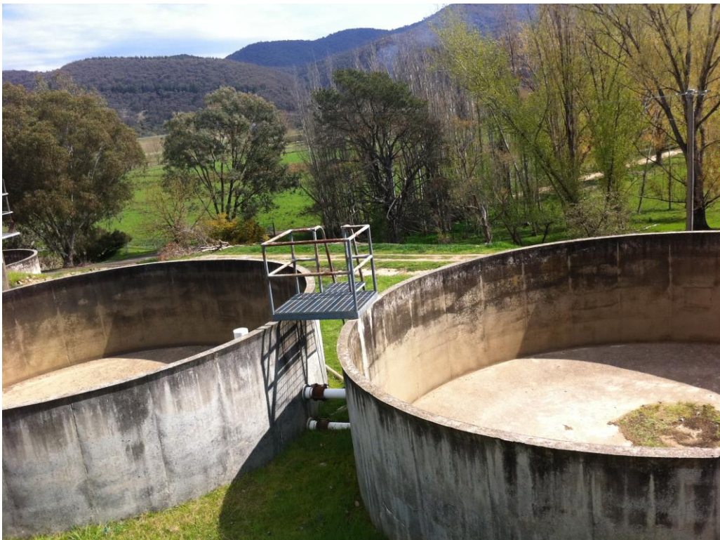
Figure 4.4 STP Stormwater Detention/ Holding Tanks
